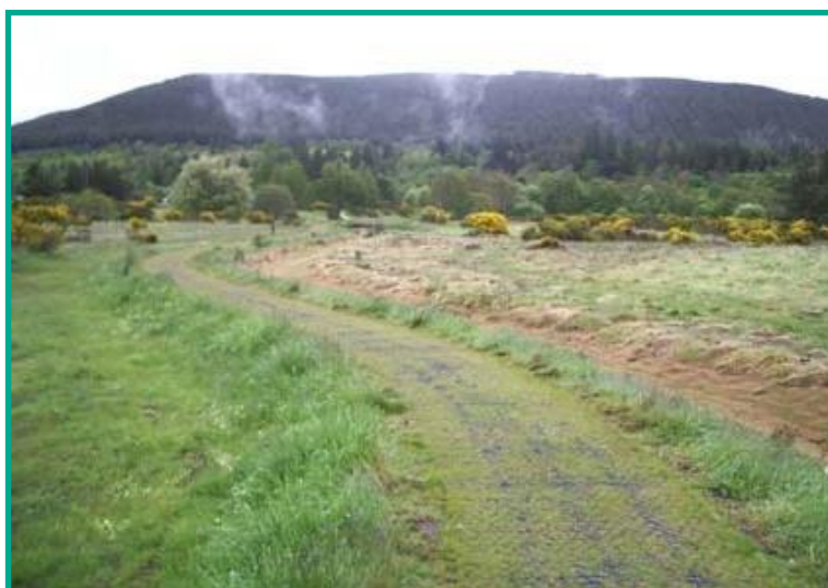
Reinforced grass path on the floodplain of River Dee SAC.
