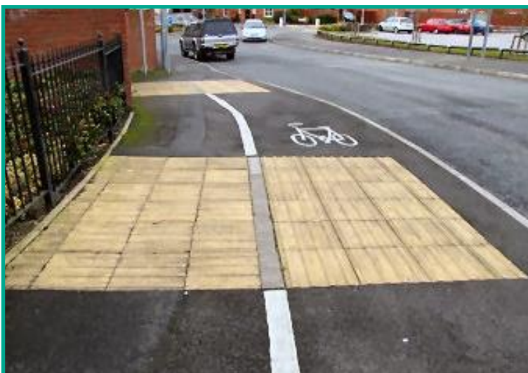
Tactile pedestrian / cycleway paving (© Paving Expert).
