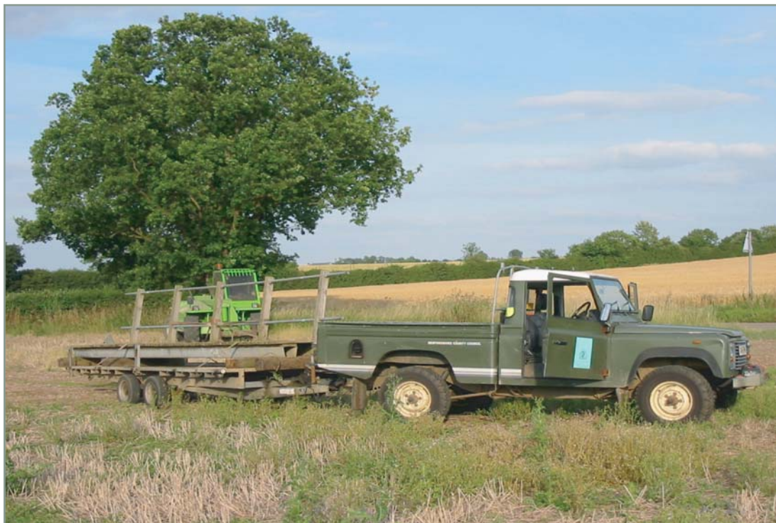
No longer needed at its present location this 7.2m footbridge was removed using a farm forklift for reuse on another of Bedfordshire's paths.
