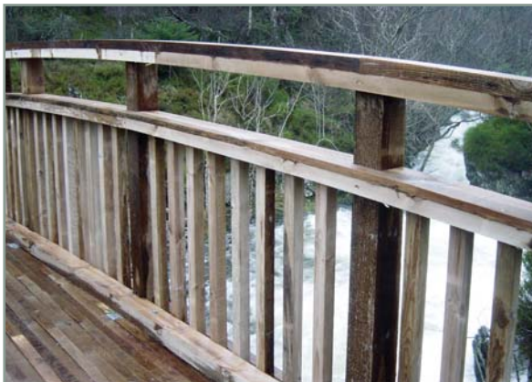
This handrail detail gives a high degree of safety for users while allowing wheelchair users and smaller people to enjoy the view
