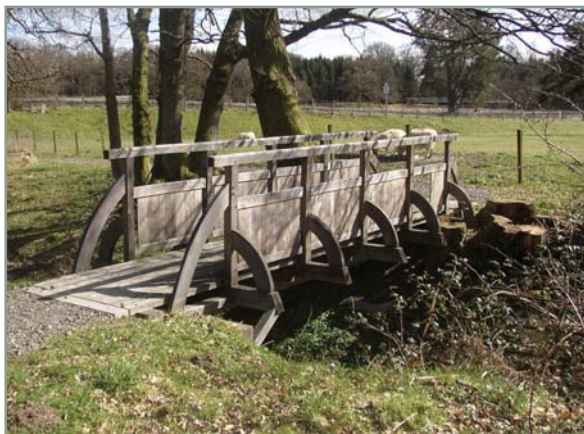
Green oak construction - a creative approach to a simply supported beam bridge
