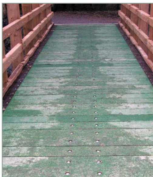
Non-slip treatment of deck boards
