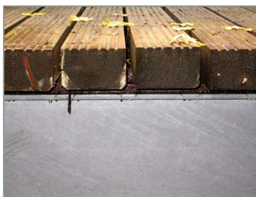
Grooved decking is available off the shelf or can be grooved in the workshop.
