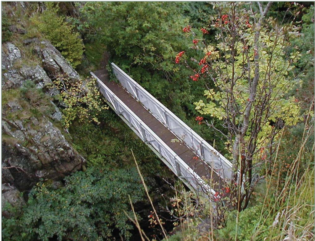
Aluminium bridge in Tillicoultry Glen. Twelve years old and no rust!
