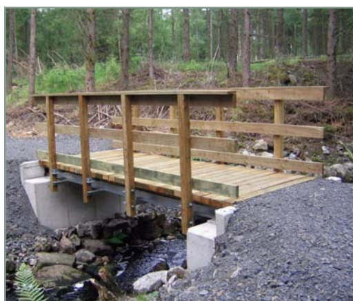
These substantial abutments are required for a short span bridge because they lie in the slip zone; the alternative would be smaller foundations and a larger span
