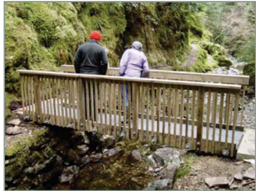
Stress laminated flat deck
