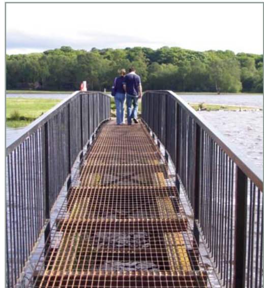
Open lattice decks can be alarming for users; dogs often refuse
