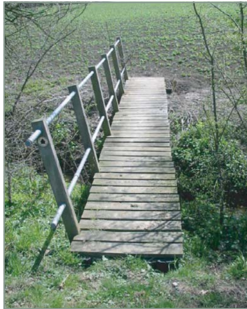
In this remote location a handrail on one side was considered adequate.
