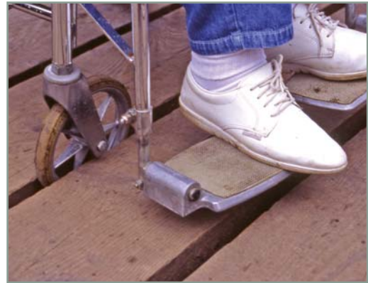
Large gaps may drain well but they are not accessible
