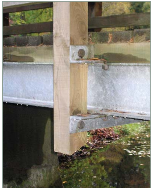
Solid post attachment on a Glentroot Bridge
