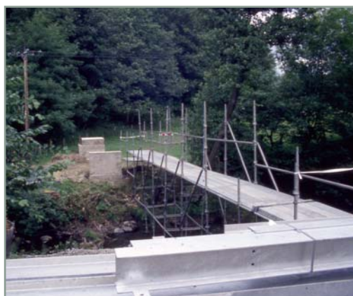
Scaffolding can allow easy access to both sides of a gap and provide a safe working platform for assembly.
