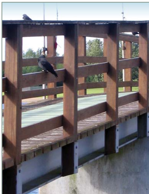
Attachments for handrail posts have been welded to the beams before galvanising
