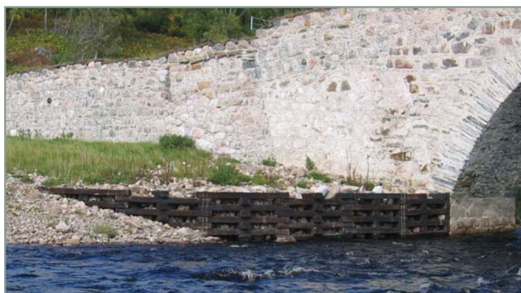
Timber revetments such as this crib wall must be robust and well constructed
