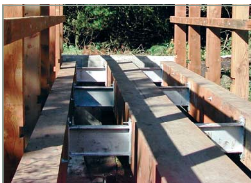
Steel bracing helps prevent both timber and steel beams from twisting
