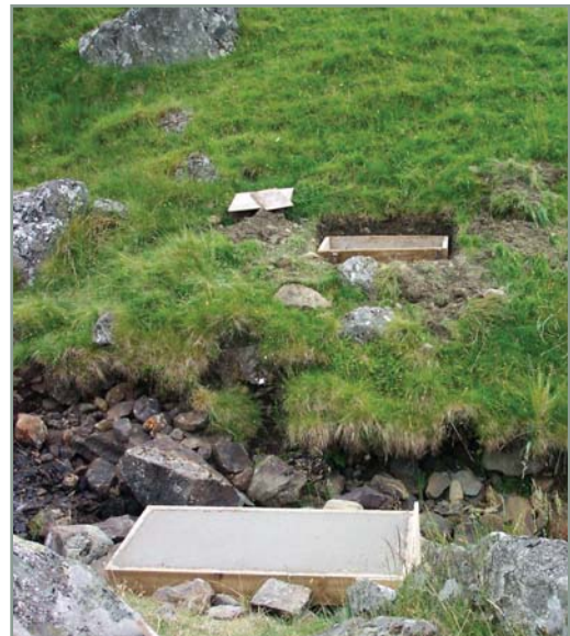
Simple concrete bankseats being formed
